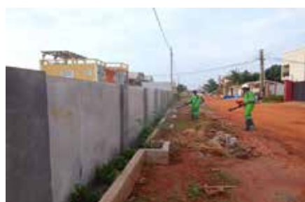
The frontage of the HR Complex which is currently undergoing beautification was not spared in the disinfection and cleaning exercise
